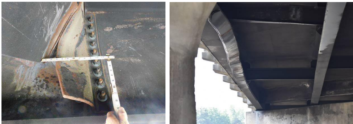
Figure A.15. Broken weld and member rotation at diaphragm [Courtesy of North Carolina Department of Transportation] and deformation in beam 4 looking south
