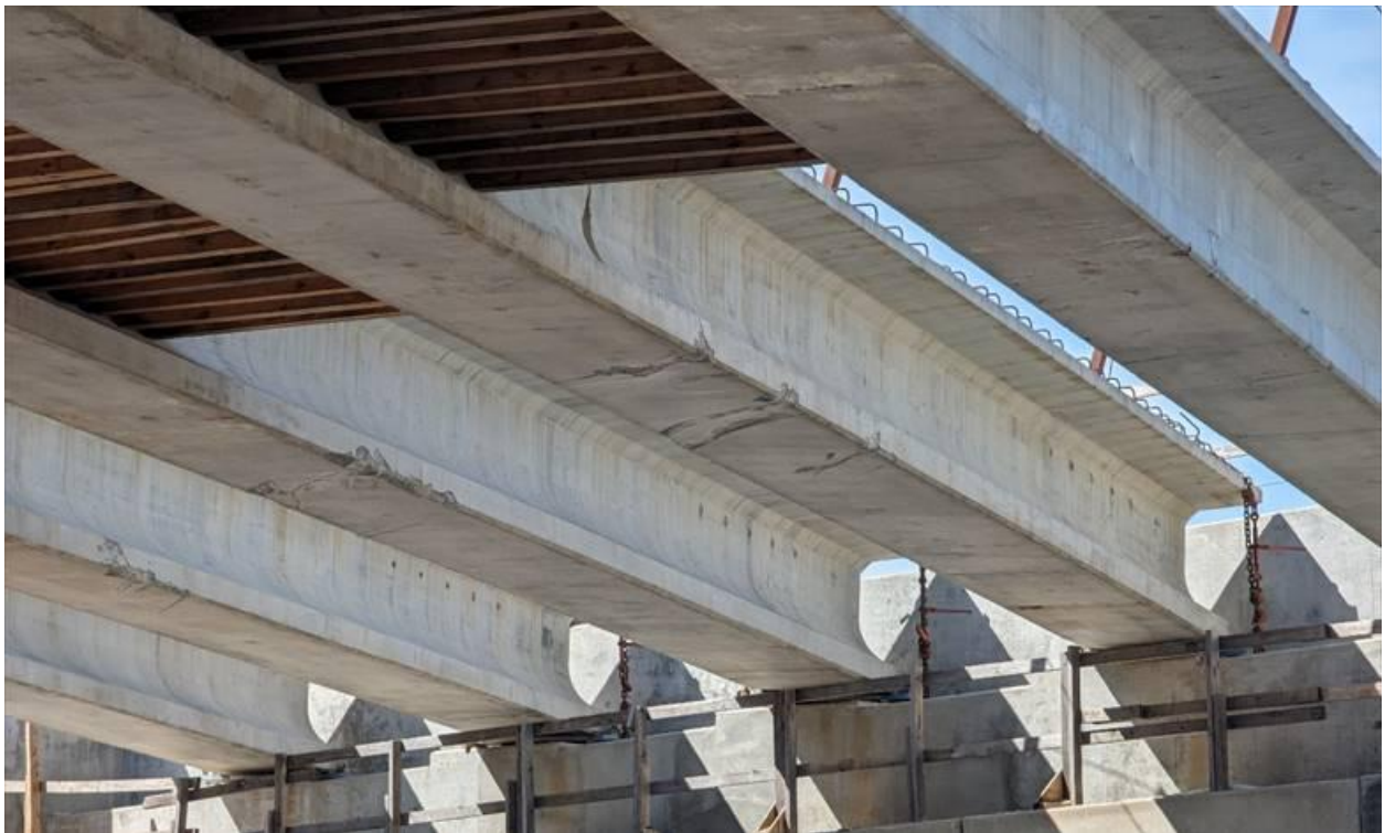
Figure A.7. Spalling and scraping at impact locations of girders 2, 3, and 4
