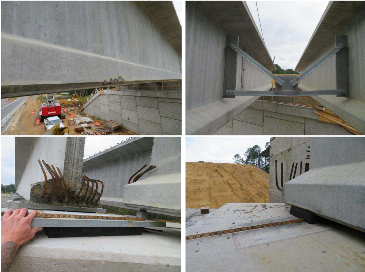
Figure A.1. Damage observed in modified bulb-tee girder of a partially constructed bridge in Wade following overheight impact [Courtesy of North Carolina Department of Transportation]
