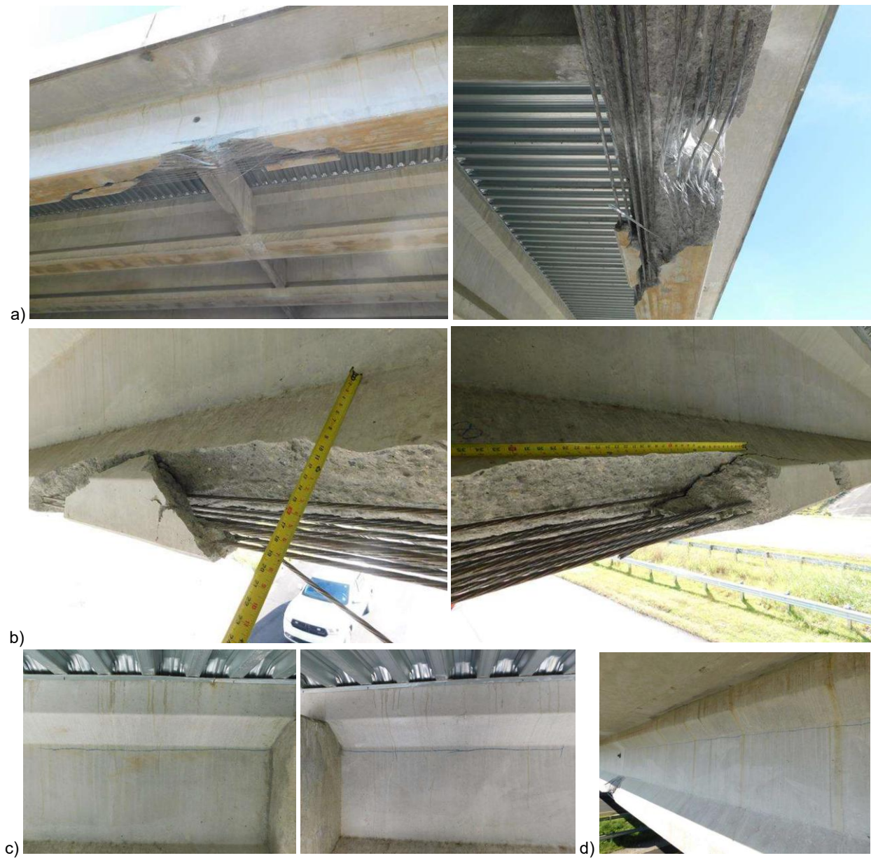
Figure A.3. Damage observed in a Greenville bridge following impact from the boom of an excavator: a) exposed and severed strands and spalling around location of impact; b) spalling across the rear side of the bottom flange; c) horizontal cracking at the web-to-top flange transition present on both sides of the intermediate diaphragm; d) horizontal cracking at the web-to-top flange transition on the impacted side of the girder [Courtesy of North Carolina Department of Transportation]
