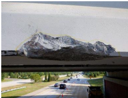
Figure A.10. Exterior girder damage [Courtesy of North Carolina Department of Transportation]
