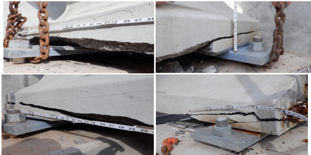
Figure A.5. Typical damage at base plate at bents [Courtesy of North Carolina Department of Transportation]
