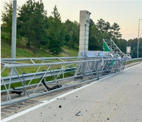
Figure A.8. Sign structure impacted and detached dump truck bed [Courtesy of North Carolina Department of Transportation]
