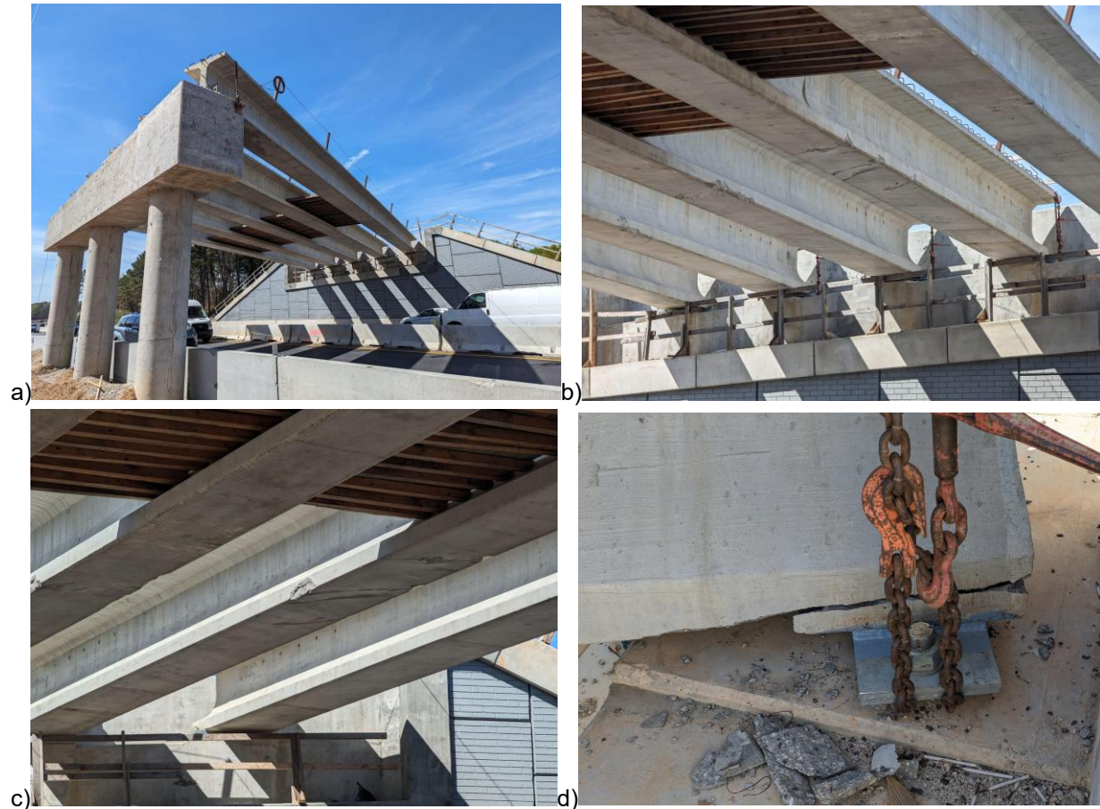
Figure 3.4. Photographs of partially constructed bridge subject to accidental overhead vehicle collision: a) status of bridge construction at time of incident; b) spalling of impacted side of bottom flanges; c) scraping of underside of girder and spalling on rear side of flanges; d) severe damage adjacent to sole plate connections
