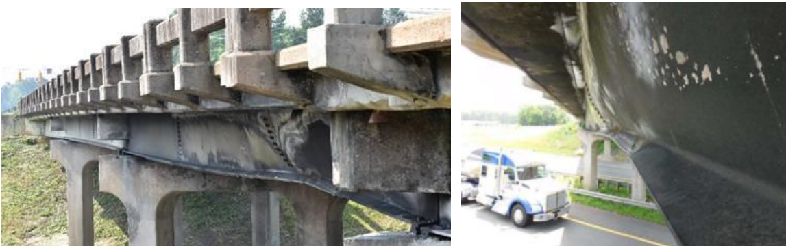
Figure A.12. Overall damage to exterior girder [right photo Courtesy of North Carolina Department of Transportation]
