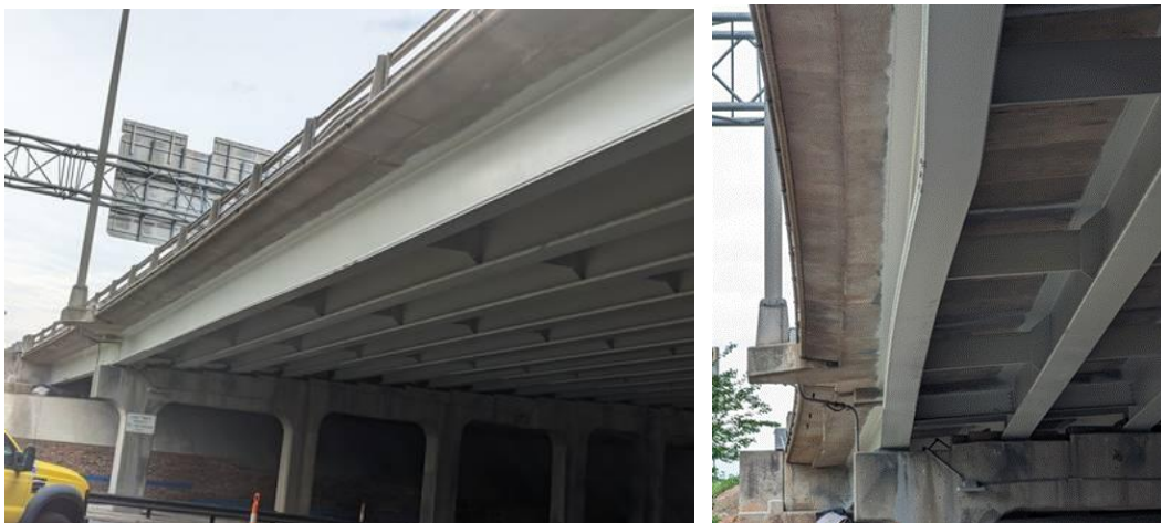
Figure A.17. View of steel girders in bridge and lateral deformation of impacted girder
