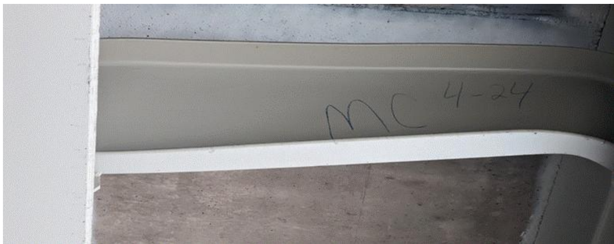
Figure A.18. Buckling intermediate diaphragm closest to impact site
