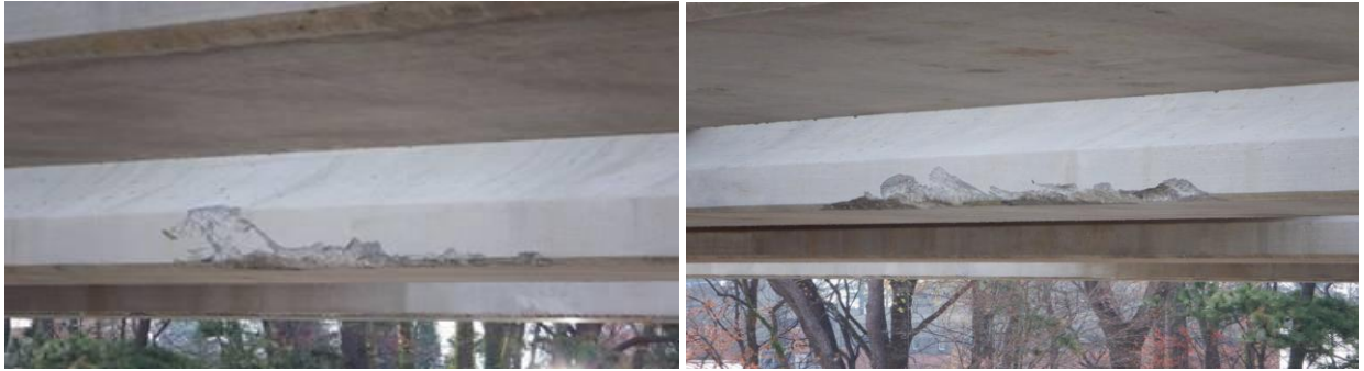
Figure A.6. Spalling at impact location [Courtesy of North Carolina Department of Transportation]
