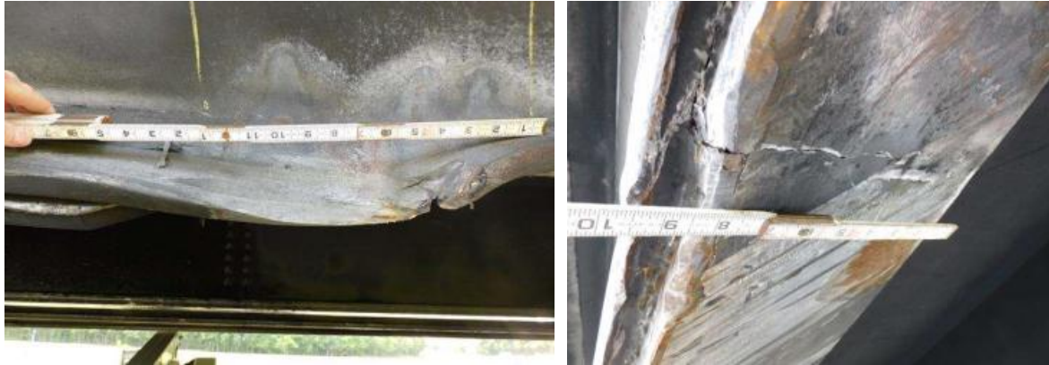
Figure A.14. Rotation and fracture at impact site. [Courtesy of North Carolina Department of Transportation]
